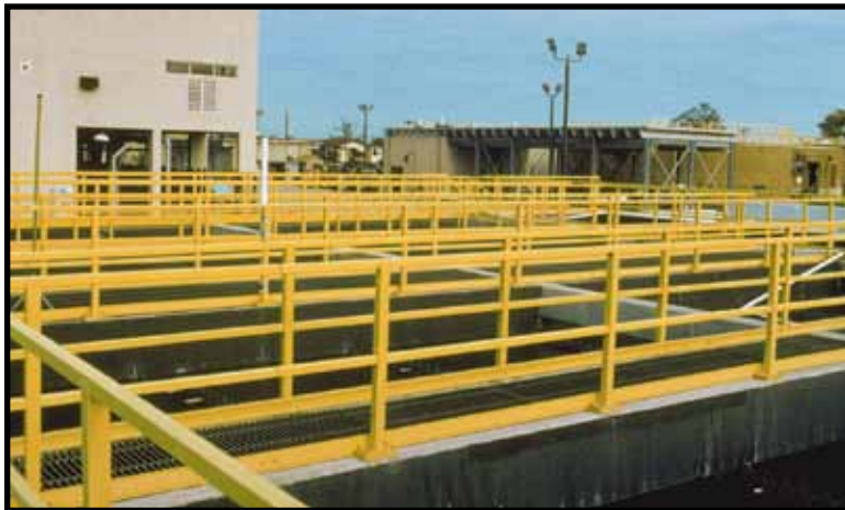
Square tube handrail manufactured with Dynaform component products offer long life in the corrosive environment of this wastewater treatment plant.
